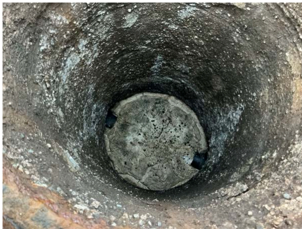
Outback Steakhouse: Outlet sample box to District line was filled with grease (before & after)
