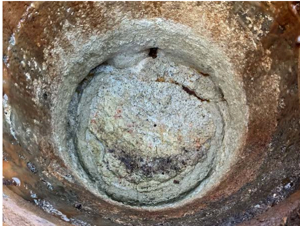
Hien Thanh Restaurant: Baffle pipe missing, system needed cleaning (before & after)
