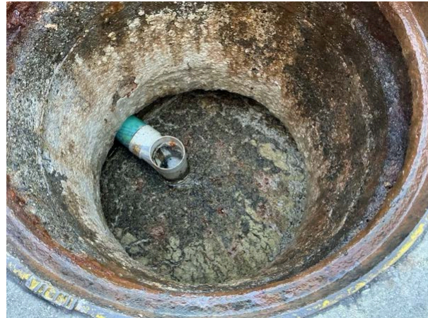
Hien Thanh Restaurant: Baffle pipe missing, system needed cleaning (before & after)
