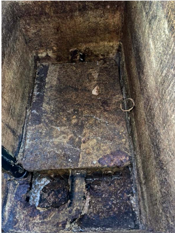
Pho Banh Mi Che Cali: Vaulted grease trap extremely dirty (before & after)
