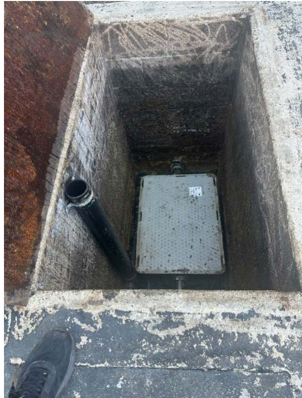
Pho Banh Mi Che Cali: Vaulted grease trap extremely dirty (before & after)
